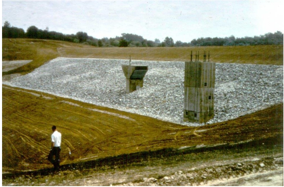
Piney Run Dam, under construction in 1974
