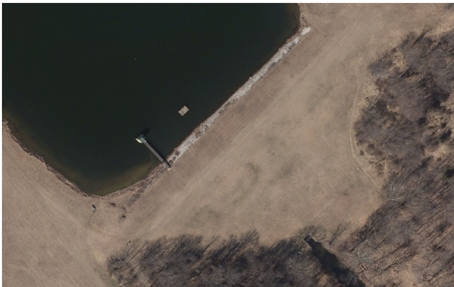
Piney Run Dam, 2017
