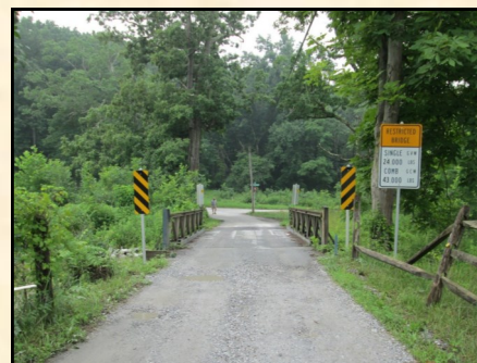
Top photo: view of Babylon Road bridge Bottom photo: looking toward Kump Station
