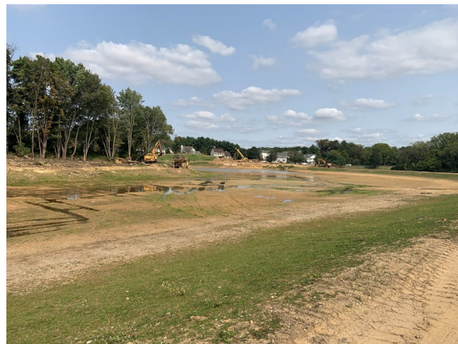
The smaller footprint of the retrofitted Willow Pond.
