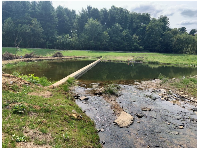
Stream channel flowing to the weir wall, where it will be diverted into baseflow to return to the stream and flood flows to enter the stormwater management facility.
