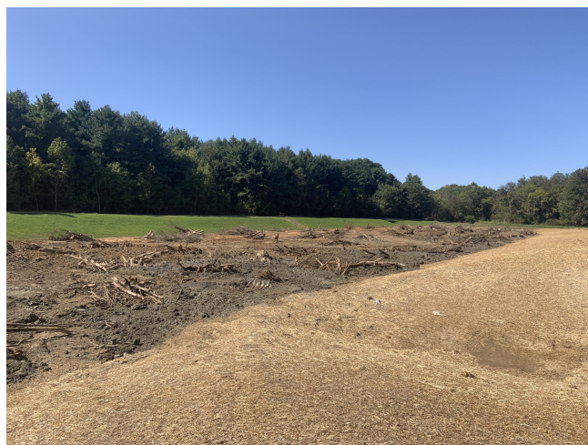
Root wads and smaller woody material being laid out for placement in localized mounded and depressional areas.
