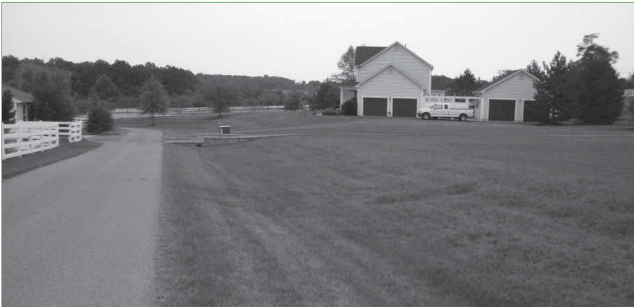
Open section roadway using wide shoulder
