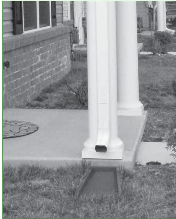
Disconnected residential downspout
