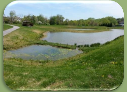
Urban Stormwater Retrofit
