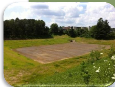
Facility at Westminster High School
