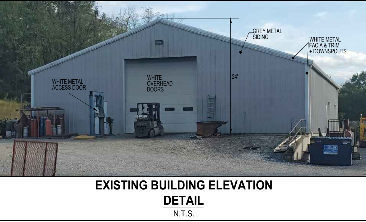
EXISTING BUILDING ELEVATION DETAIL N.T.S.
