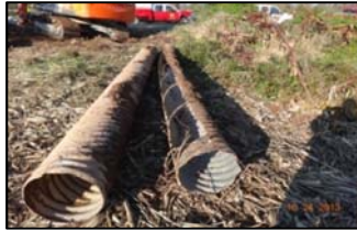
Photograph of a deteriorated metal pipe.
