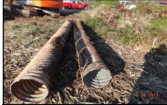
Photograph of a deteriorated metal pipe.
