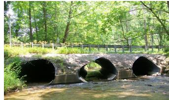
This project provides funding to replace the three cell structural plate pipe culverts, located near Finksburg, with a new structure. The type of replacement structure will be determined based on an alternatives analysis.
