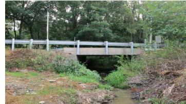
This project provides funding to replace the small bridge, located in western Carroll County near the Town of New Windsor. The existing structure is concrete encased steel beams on stone masonry abutments. The type of replacement structure will be determined based on an alternatives analysis. The structure width and waterway opening will be evaluated as part of the analysis.
