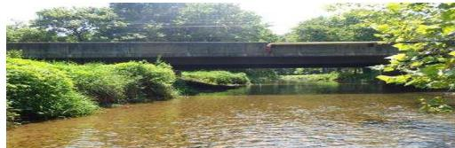
This project provides planned funding to replace the bridge, located near Mount Airy. The existing structure is a steel beam bridge on concrete abutments and pier. The type of replacement structure will be determined based on an alternatives analysis. The structure width and waterway opening will be evaluated as part of the analysis.
