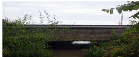
This project provides funding to replace the small structure, located near New Windsor and Union Bridge. The existing structure is a concrete slab on stone masonry abutments. The type of replacement structure will be determined based on an alternatives analysis. The structure width and waterway opening will be evaluated as part of the analysis.
