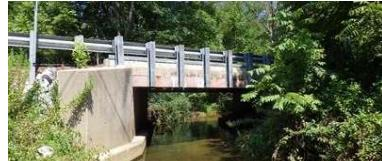
This project provides planned funding to replace the small bridge, located near Finksburg. The existing structure consists of steel beams on a combination of stone masonry and concrete abutments and wingwalls. The type of replacement structure will be determined based on an alternative analysis. The structure width and waterway opening will be evaluated as part of the analysis.
