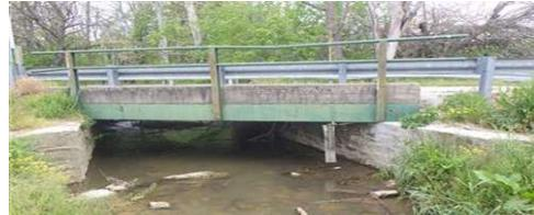
This project provides funding to replace the small bridge, located in western Carroll County near Union Bridge. The existing structure is steel beams on stone masonry abutments. The type of replacement structure will be determined based on an alternatives analysis. The structure width and waterway opening will be evaluated as part of the analysis.
