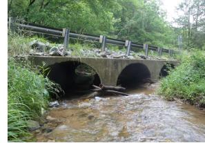
This project provides planned funding to replace the three cell corrugated steel pipe culverts, located near Finksburg, with a new structure. The type of replacement structure will be determined based on an alternatives analysis.
