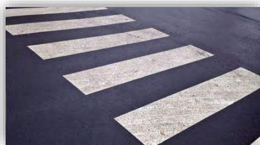
Figure 6-3: Block pattern crosswalk
