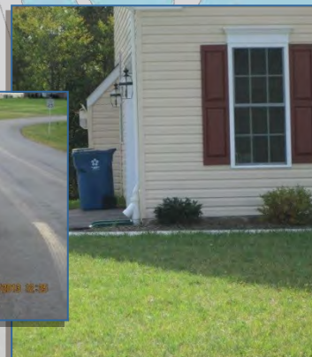
Residential: Drywell with Debris Filter
